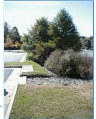
Example of a biofilter installed to clean parking lot runoff
